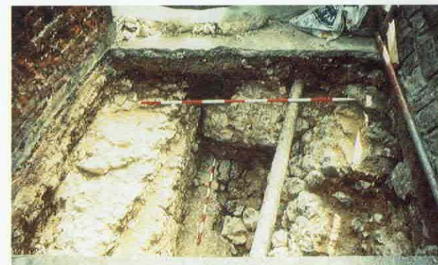
The footings of the original 12th century stone keep on the motte of Windsor Castle: to the right, the battered flint plinth of the first keep surmounted by the hearthstone plinth of the second keep; to the left the medieval mantlet wall topped by the thinner 17th century parapet of the Carronade. © EH.
