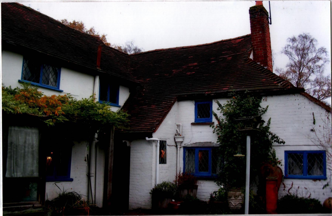
SE Side View from the rear. Phase 1 to the right, phase 2 to the left looking N
