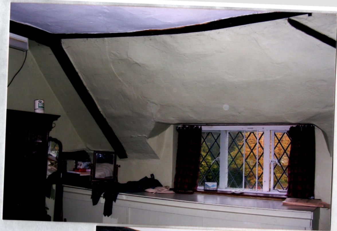
Bedroom 1st floor of hall looking NE
