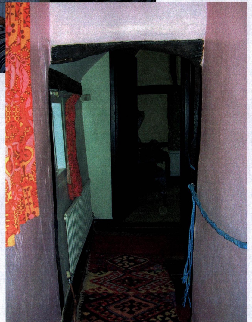
Looking NE from phase 2 into cross-wing. Upper curved timber marks end wall, cut through for access.
