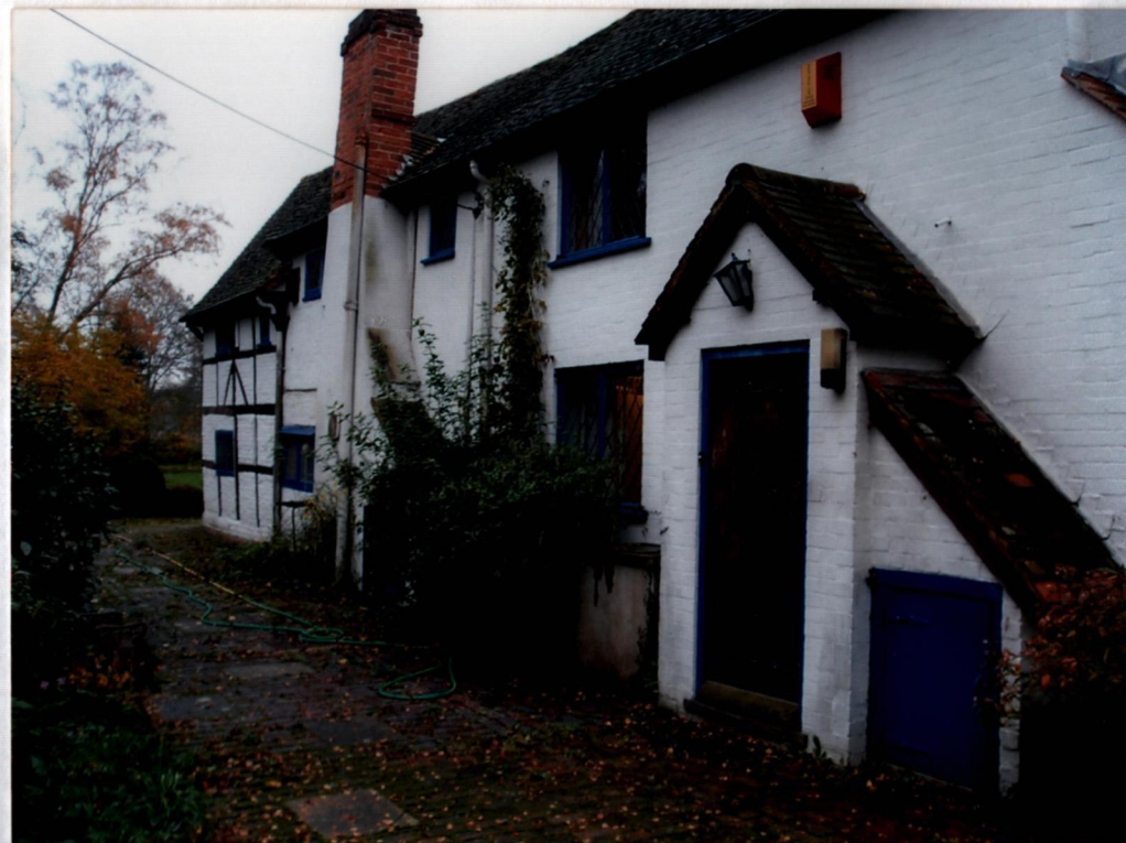
Along front extension to original part
