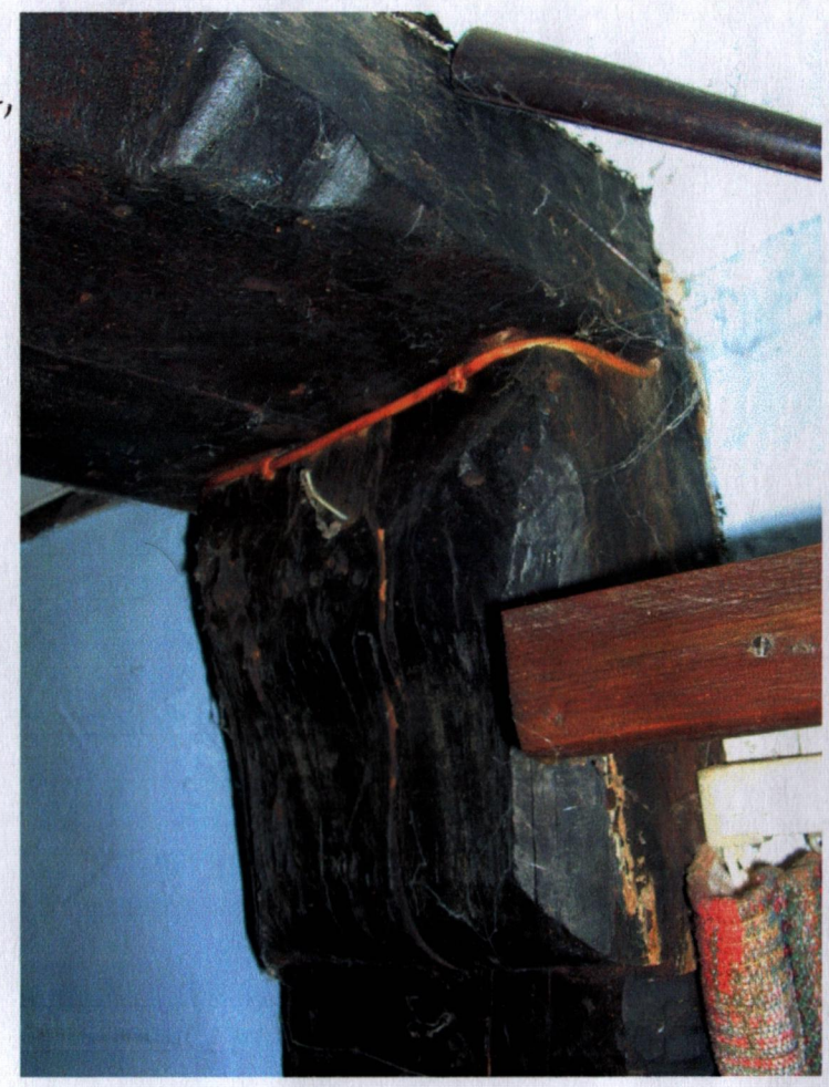
Ogee stop on transverse beam
