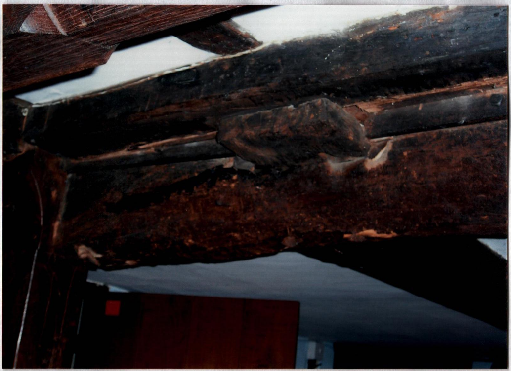
Looking NE from phase 2 (with cross wing) upper curved timber marks end wall, cut through for access
