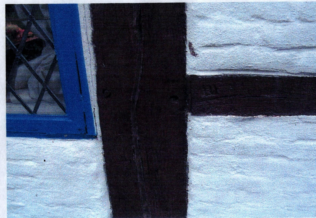
Exterior: carpenter's mark detail
