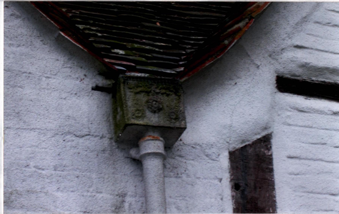
Rainwater hopper at junction of the gables
