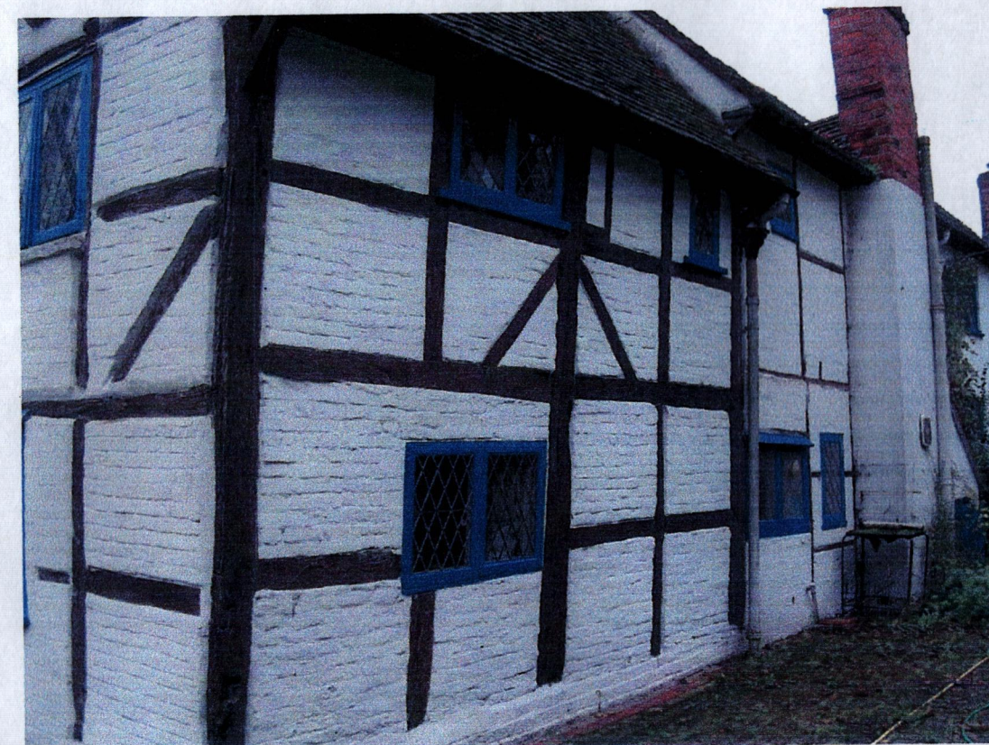
Exterior : NW side
