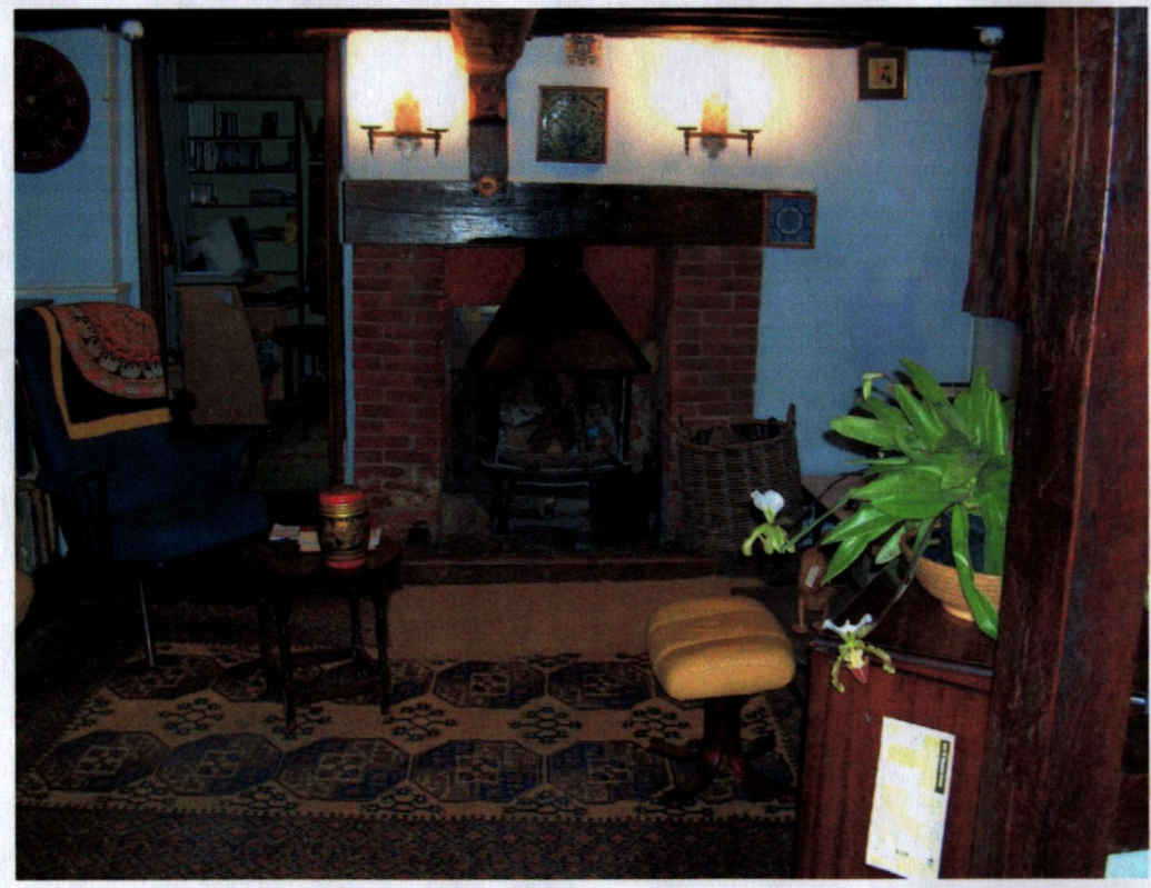
Ground floor looking SE. Axial beam is visible top centre, with joists off to left and right, and inserted fire place ahead.
