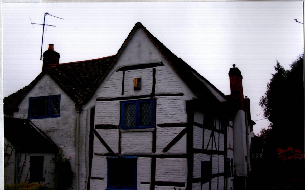
Oldest part on N.W. Corner
