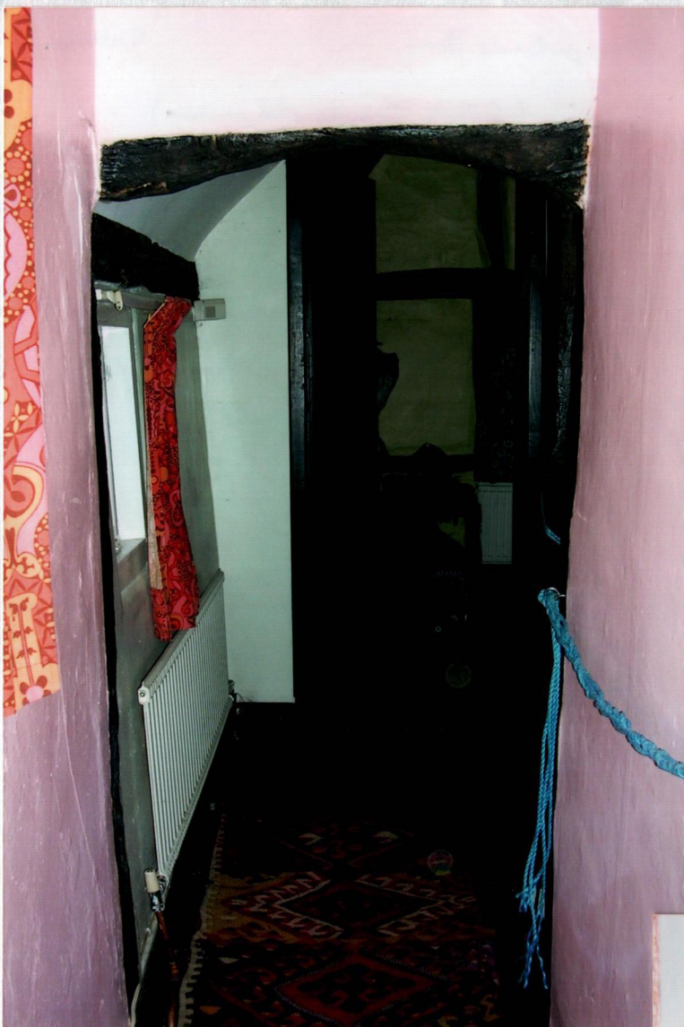
Looking NE from phase 2 (with cross wing) upper curved timber marks end wall, cut through for access
