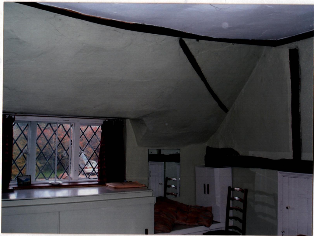
1 st floor of hall, looking NE (window looking towards garage)
