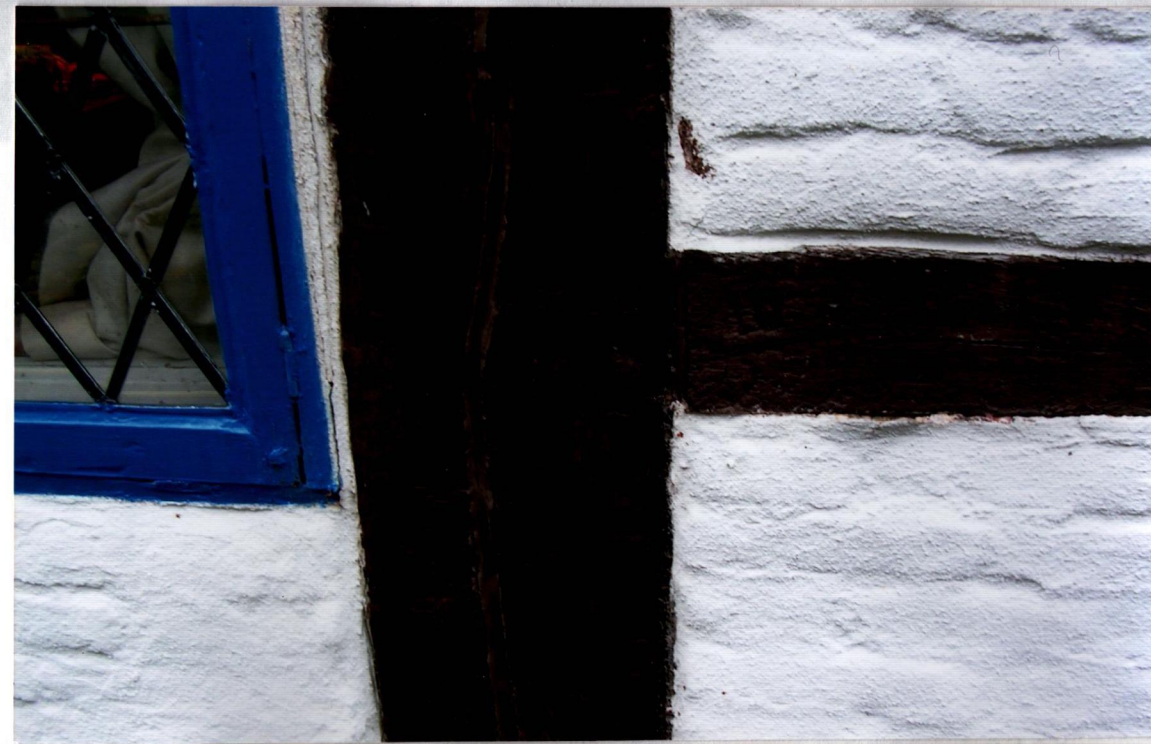
Exterior detail Carpenter's mark.
