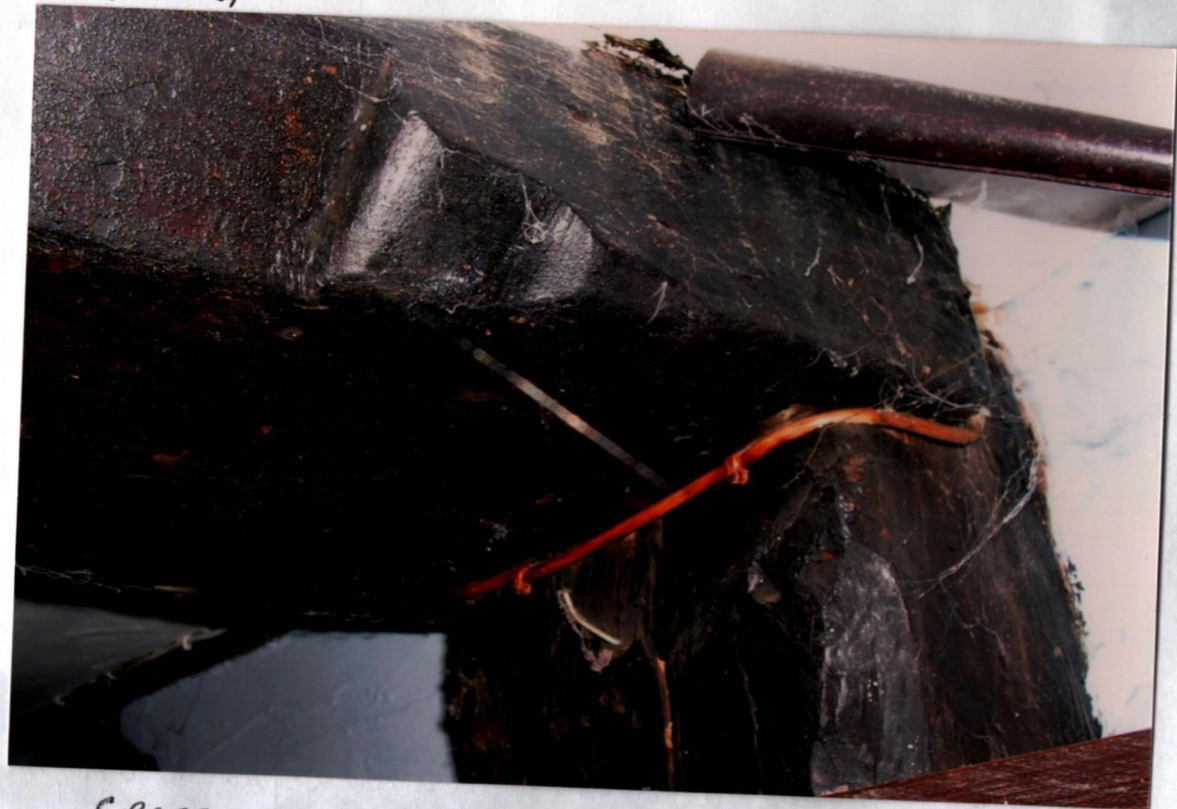
Crossing NW side Towlea Post. Ogee stop on Transverse beam
